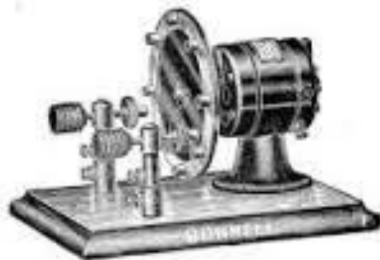
ROTARY SPARK GAP.
