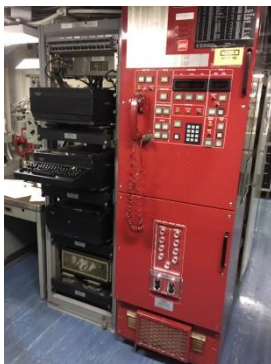
SA-2112(V)4/STQ Switching Matrix (Coke Machine)
